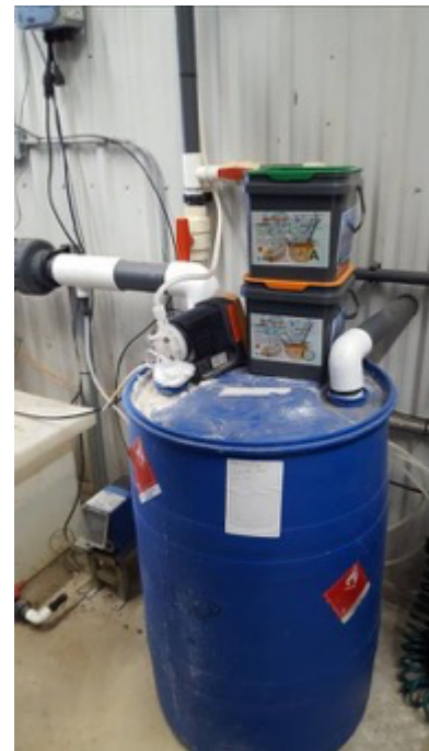
Figure 4.7 ClO 2 injector system
