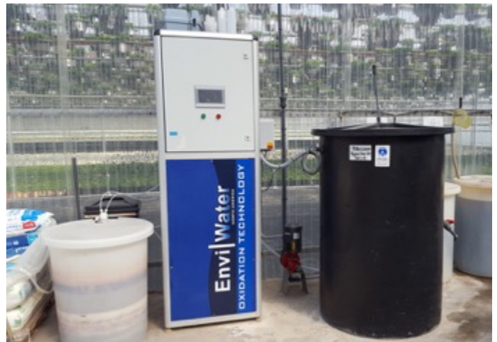
Figure 4.8 Electro-chemical-activation (ECA) system
