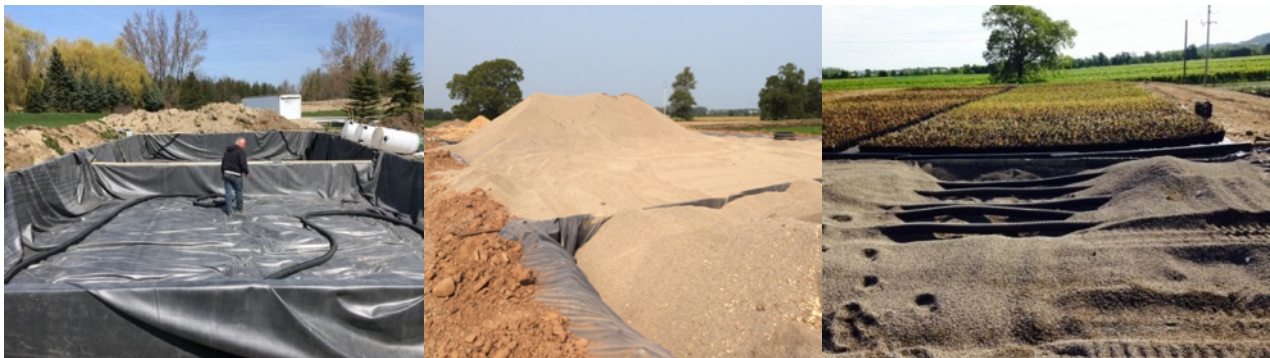
Figure 4.20 Installation stages of HTS, showing lined cell preparation, media (woodchips in back, filter sand and pea gravel to the front) and potted plants set on top.
