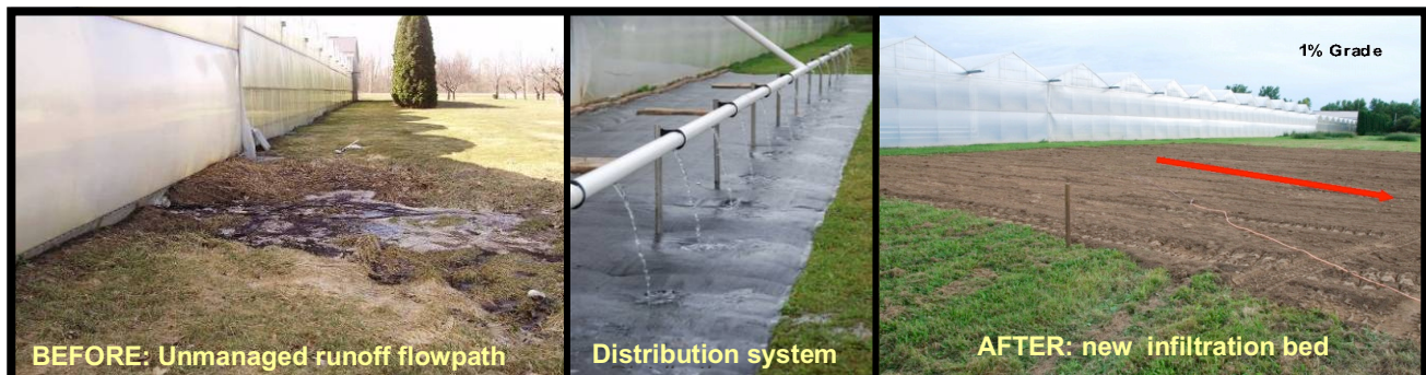
Figure 4.28 Before and after installation of a VFS at a greenhouse facility; close-up of distribution pipe
