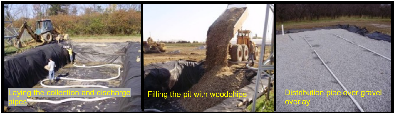
Figure 4.19 Construction of a woodchip denitrification bioreactor at a flower greenhouse operation
