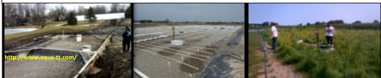
Figure 4.15 Subsurface vertical flow wetland (construction and mature wetland; Aqua Treatment)
