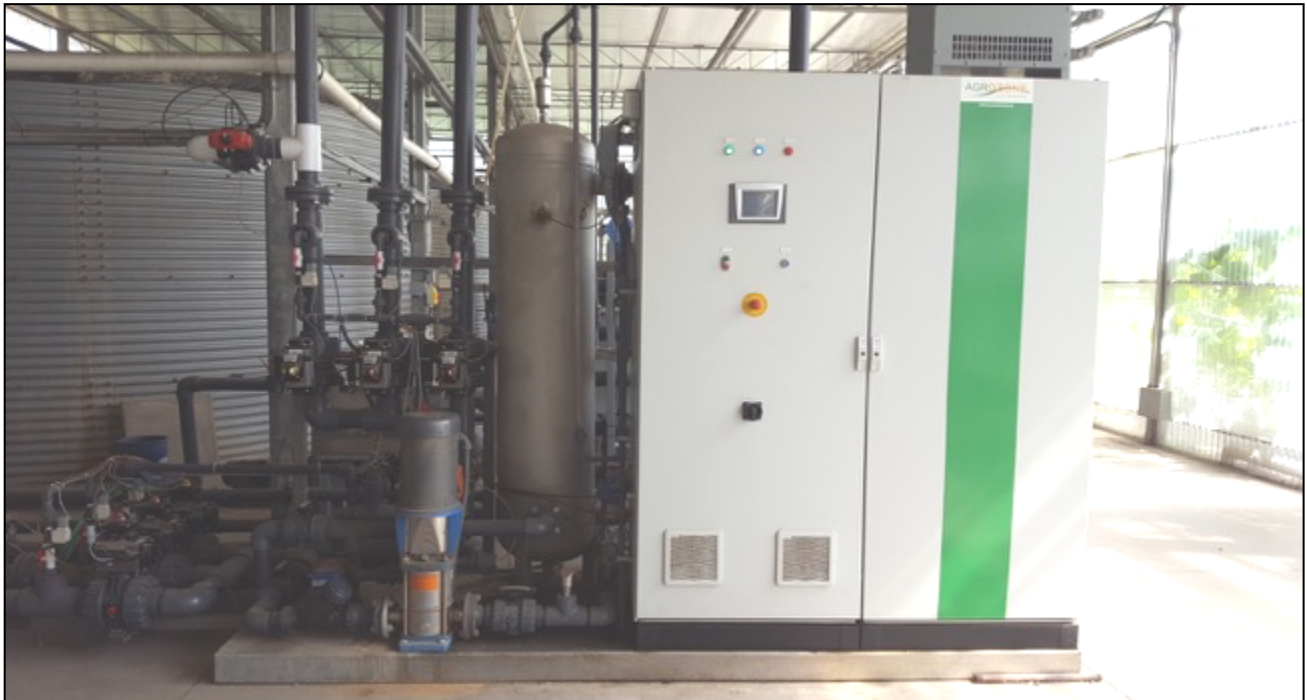
Figure 4.10 Ozone system installed at a vegetable greenhouse
