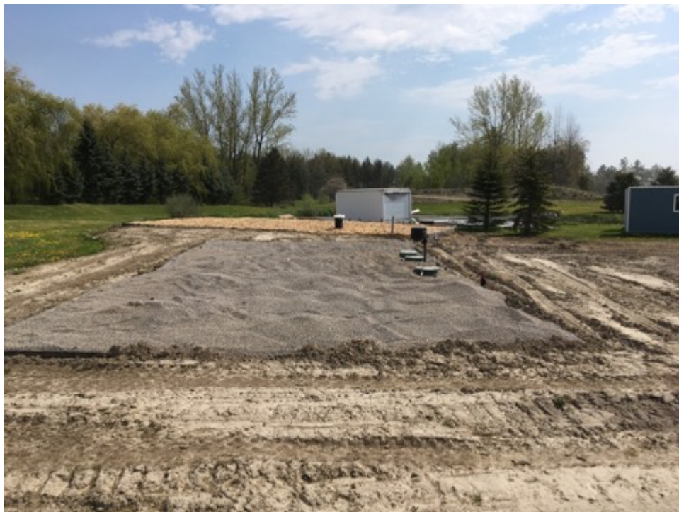
Figure 3.1 Hybrid Treatment System with woodchip cell in the background, and pea gravel and filter sand cells in the foreground.
