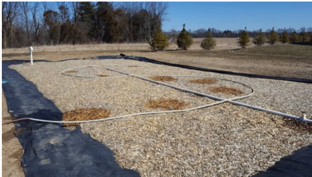
Figure 3.3 Woodchip Denitrification Bioreactor
