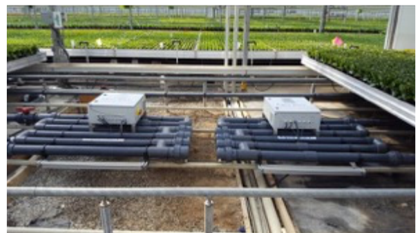
Figure 4.11: Copper Ionization systems (Aqua-Hort), vertical and horizontal under bench installations
