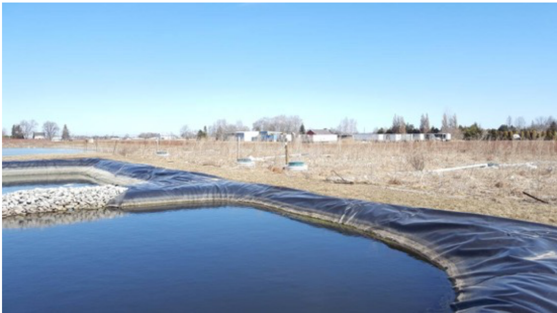
Figure 3.4 Settling Ponds and Constructed Wetland
