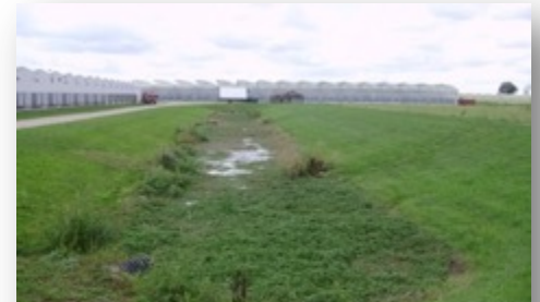
Figure 4.25 Bioswale to manage roof stormwater runoff. The vegetation consists mainly of naturally developed water cress bed.
